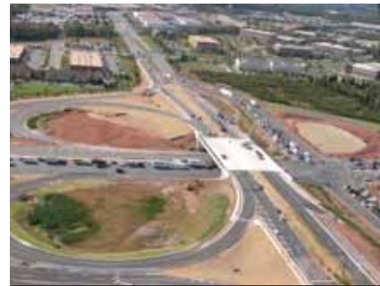
Jurors awarded the Route 28 Interchange Improvement project team the transportation and structures top award for "making things easier for the client."
